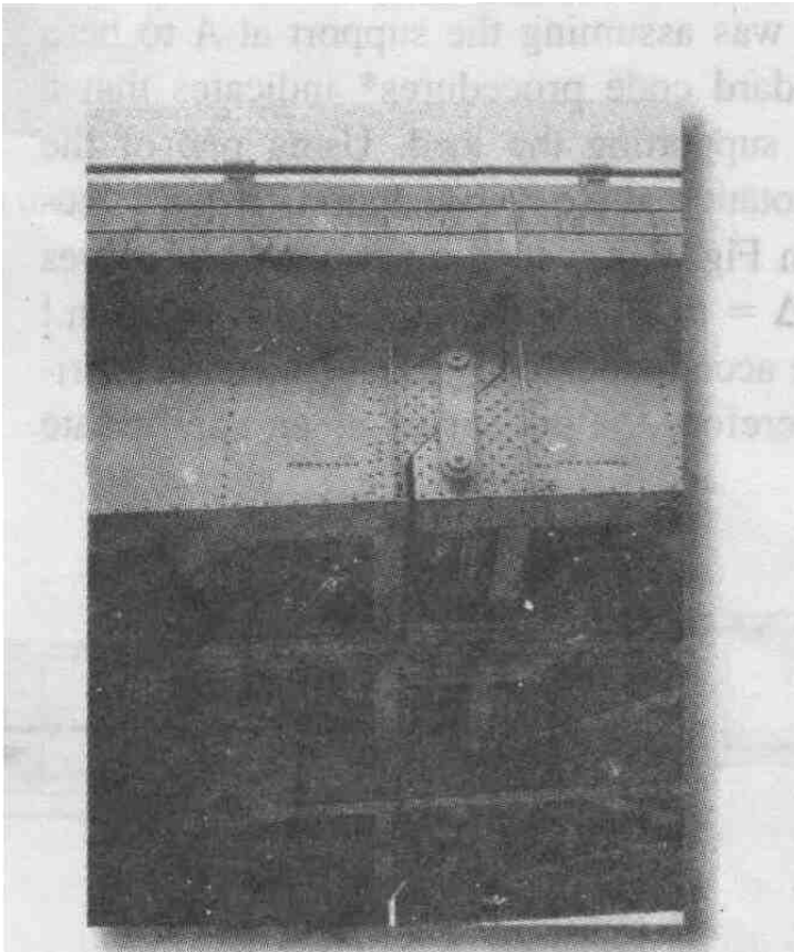
The short link is used to connect the two girders of the highway bridge and allow for thermal expansion of the deck.
