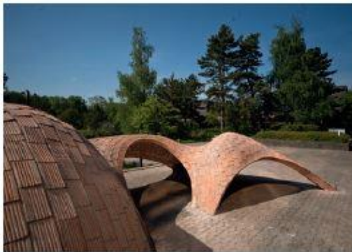
Figure 7.1 Tile vault prototype at ETH Zurich, Switzerland, 2011
